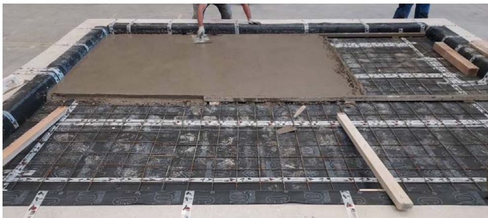
Photos of assembly of test specimen
