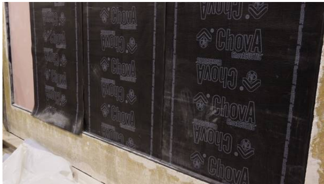
Photos of mounting of wall lining
