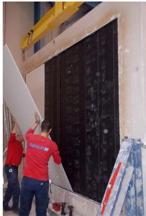
Photos of mounting of wall lining
