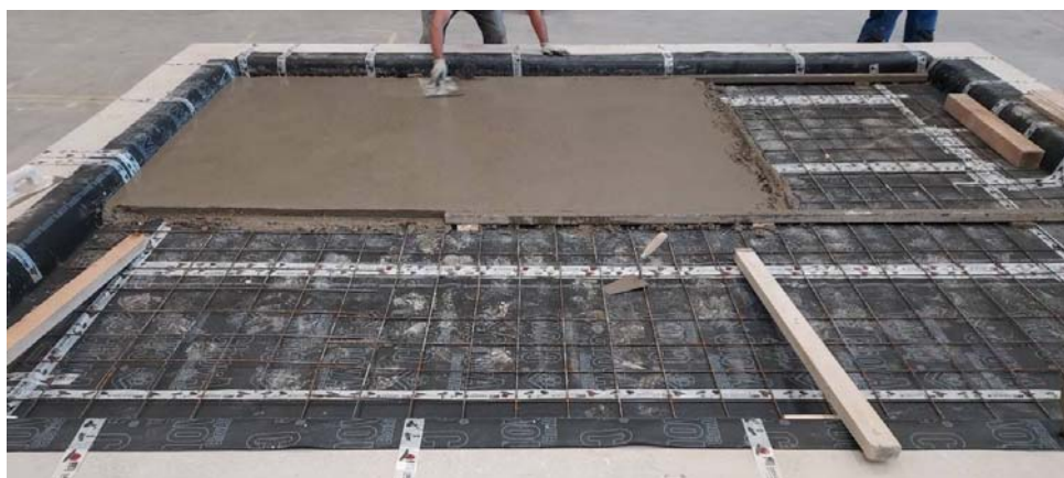
Photos of assembly of test specimen
