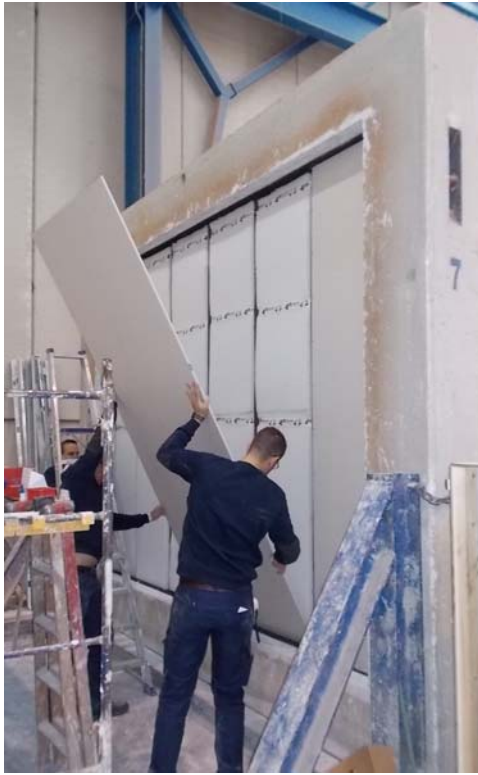
Photos of mounting of lining
