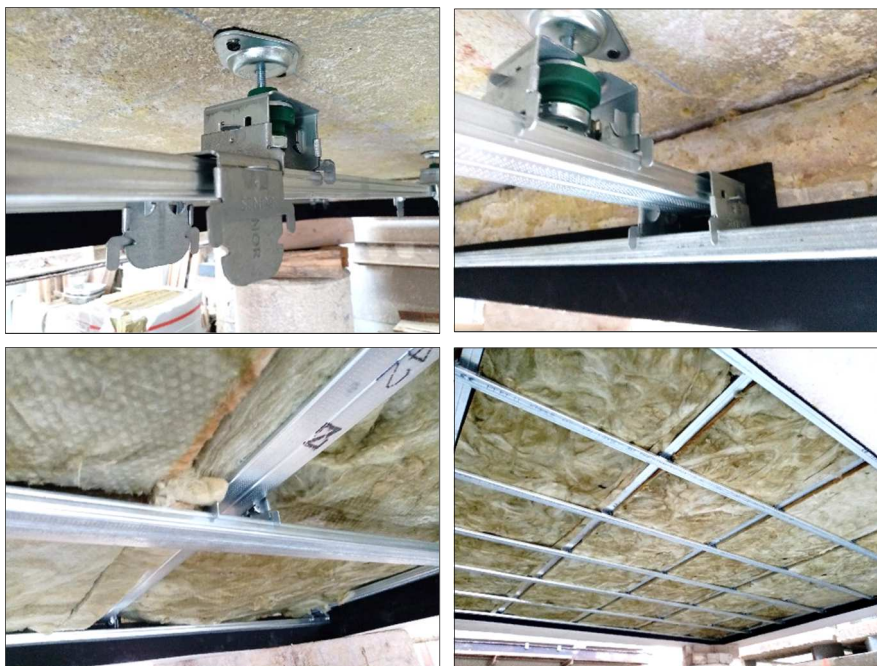
Images 16 to 19 Structure and mineral wool installation
