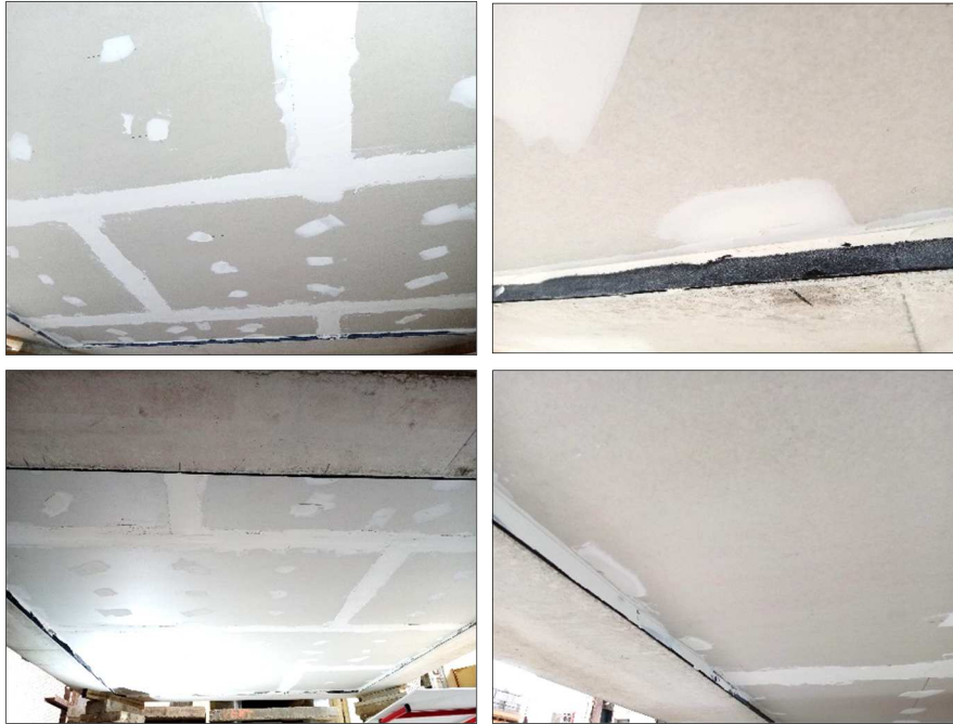
Images 20 to 23 Installation and sealing of 1 st layer of plasterboard
