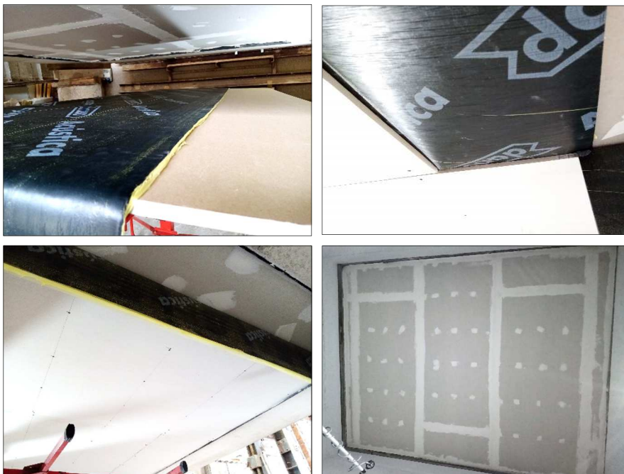
Images 24 to 27 Bituminous membrane and 2 nd layer of plasterboard installation
