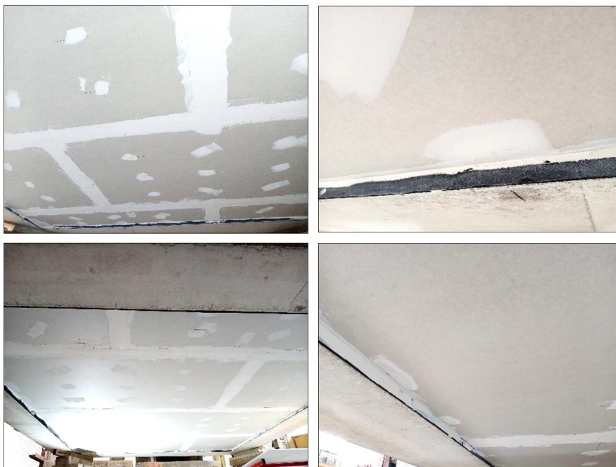
Images 18 to 21 Installation and sealing of plasterboard
