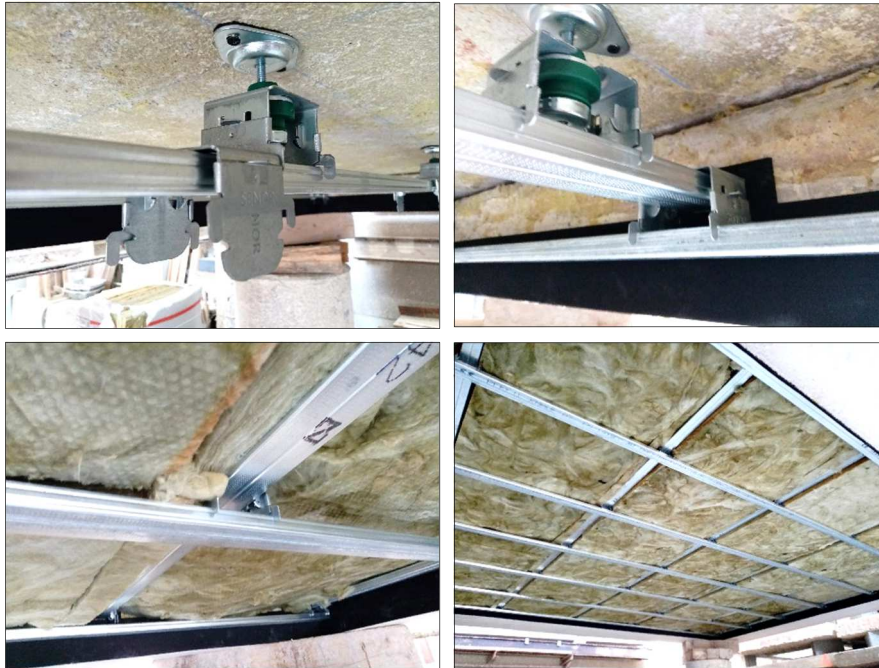
Images 14 to 17 Structure and mineral wool installation
